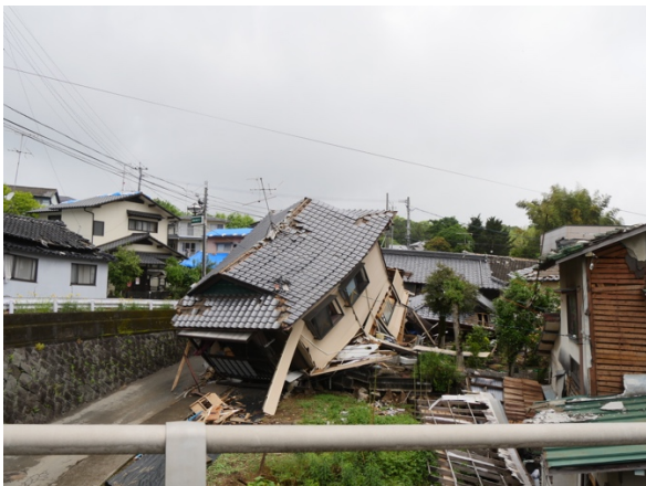
Destroyed and damaged Houses
